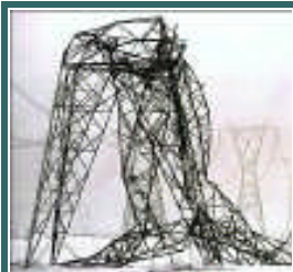
Ice storm crushed power distribution system in China.
